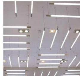
**LIGHTING RETROFITS IN SAN FRANCISCO** maximize efficiency and save on site costs. New LED lamps along with “Smart” light technology provide annual cost savings of \$124K and are expected to generate \$618K of savings over the next five years.
